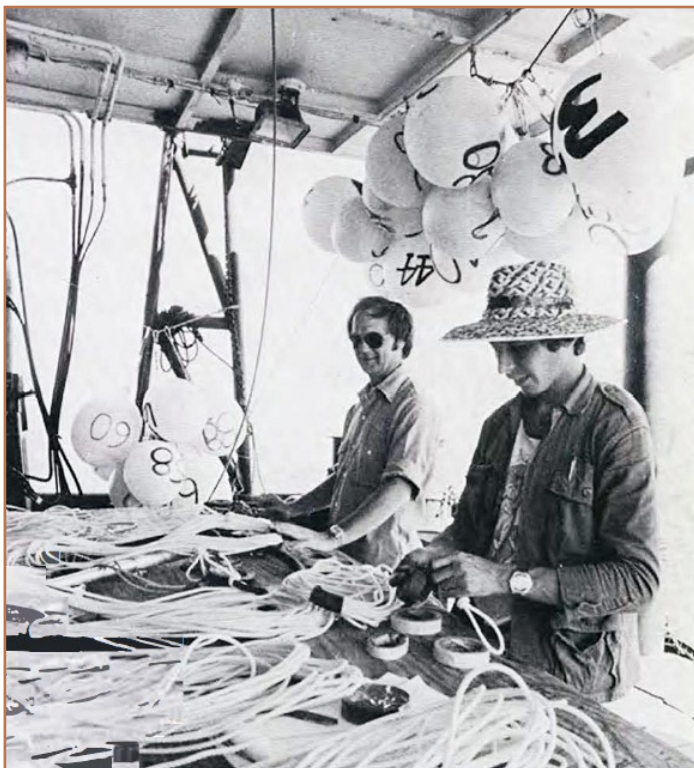
Figure 2: Field Supervisor Dave Durham (left) and Helper Paul Best are working with Party 181 on the Western Beach offshore Egypt in the Red Sea as they cut ropes to specific lengths for the navigation buoys.
