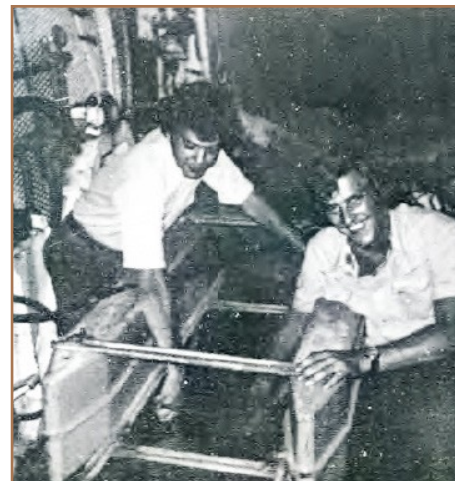
Figure 5: Party 76 Helper William "Bill" Regone (left) and Junior Observer Peter Van Borssum prepare to launch a Uni-Boom sled and a transducer from the Western Gulf, which is working in the Gulf of Mexico.
