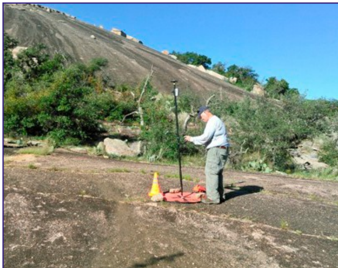
Figure 2. Raptor Aerial Services fixes a GPS location at the base of Enchanted Rock to calibrate the follow-on drone topography survey.
