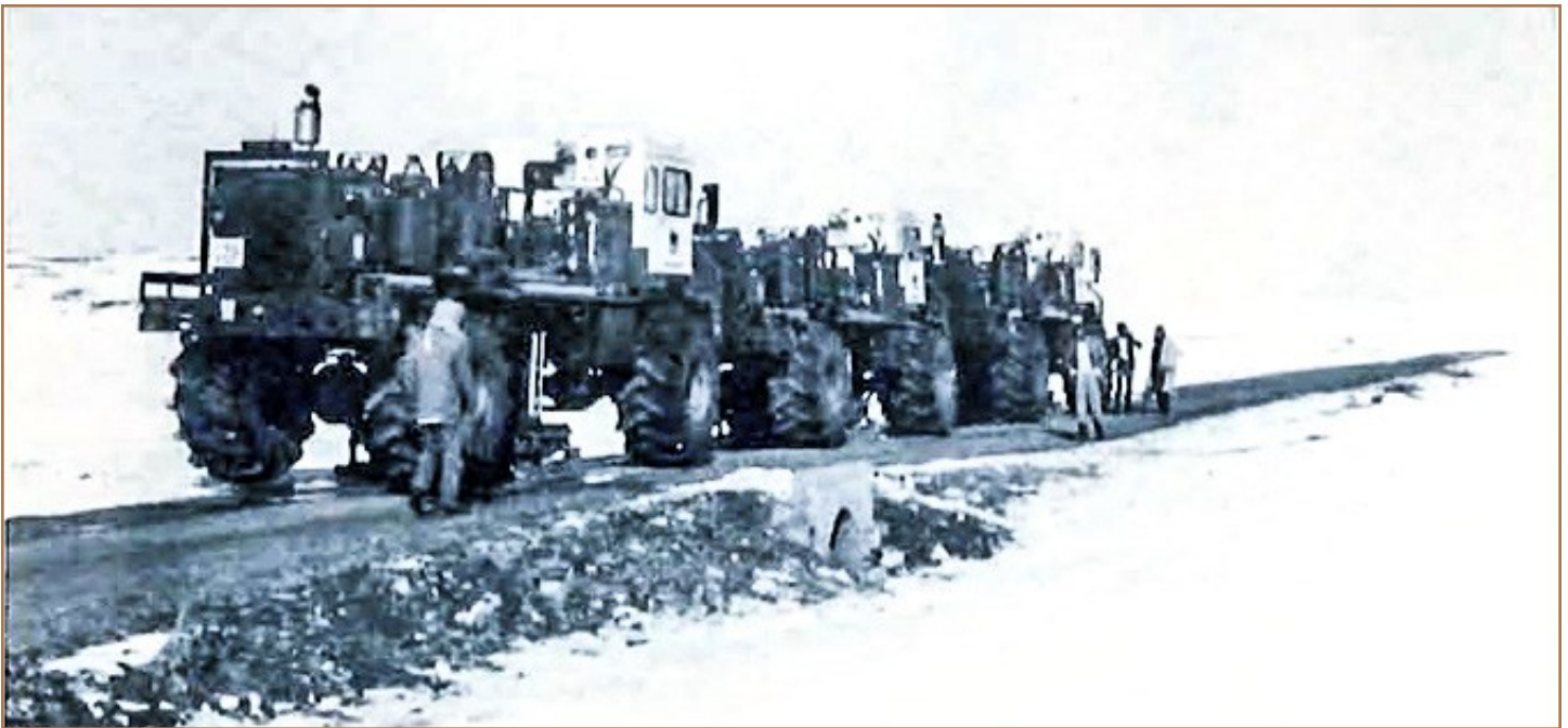
Party 1620's TR-4 vib trucks on line and getting ready to record a shot. Note that the first vib truck is lifted in the air being supported by its vib plate as it goes through its tests.
