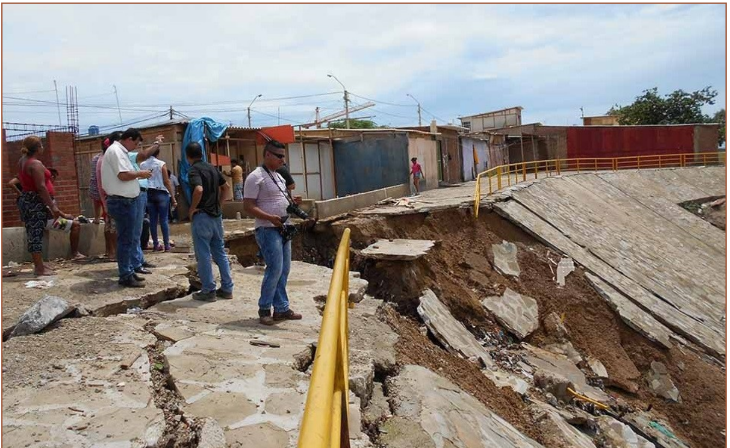
Figure 6: Damage to existing infrastructure as a result of the floodwaters. Photo credit: El Regional Piura
